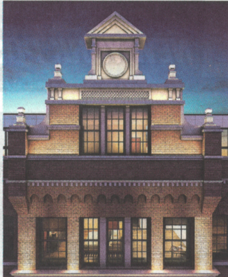
A new light installation at The Schumacher (36 Bleecker St.) spotlights the building's rebuilt pediment crown.
